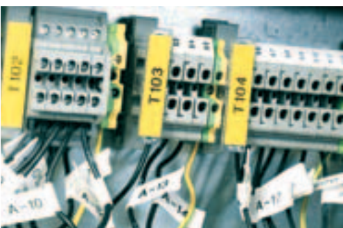
Any manufacturer brand of terminal blocks can now be marked fast with one long label.
